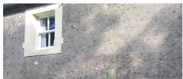
Smooth render lined out to imitate stonework
