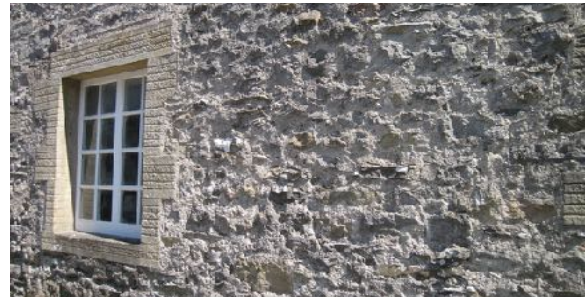
Flush pointing limestone
