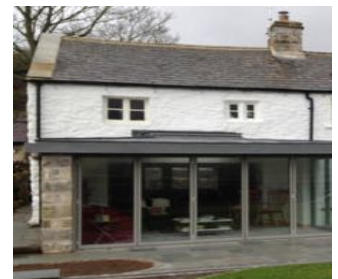
zinc roof to extension (Austwick)
