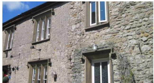
Left - lime roughcast render & sash windows Right - rubble stonework & casement windows
