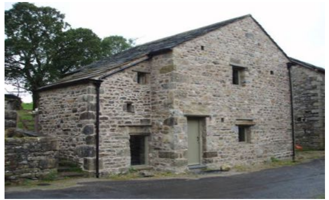
Windows set back with grey/green paint finish
