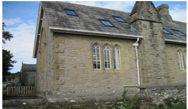
Semi dressed and coursed gritstone with sandstone dressings
